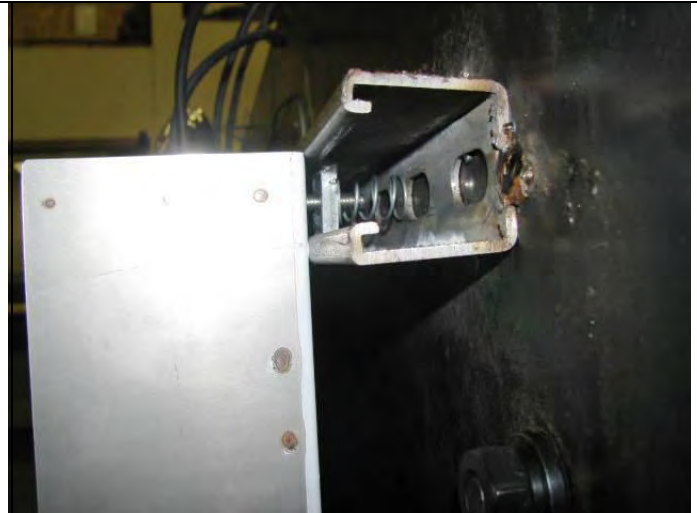
4726 ELU S/N 100013 Unistrut mounting hardware 3 places, Torqued to 78.5 in/lbs.
